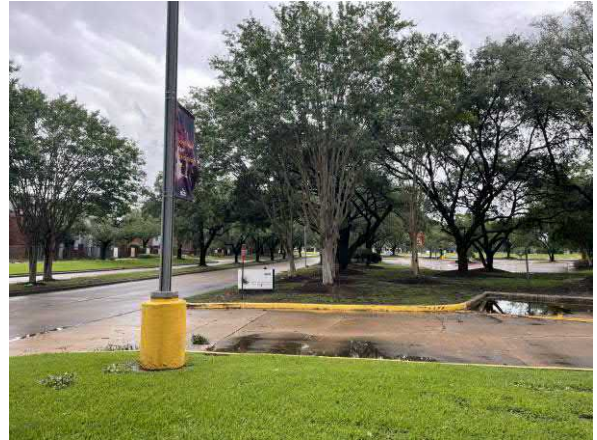
Photo 2 View of the northern boundary of the site facing east
