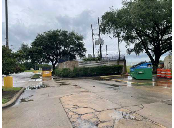
Photo 14 View of the on-site dumpsters and chiller enclosure area
