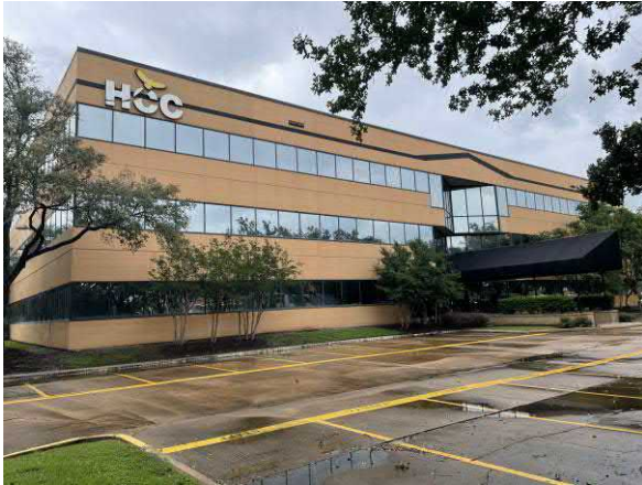
Photo 1 Typical view of the site
