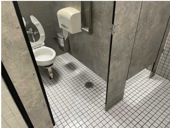
Photo 9 Interior floor drain within an on-site restroom
